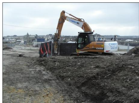
Construction of the new bridge over the west end of Copperhouse Pool, necessitated construction of a temporary causeway and piling into the riverbed. This required careful planning and mitigation to avoid poor water quality, disturbance to the birds feeding and resting on the pool flats, effects on the fish and saltmarsh in the pool, and alteration of the tidal regime in the pool. Careful restoration of the shore was essential once the temporary causeway was removed.
